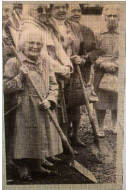
Fellowship Hall Groundbreaking
